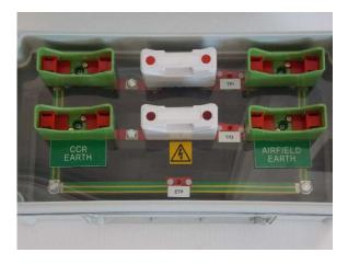
In the normal position (white links in centre white holders) electrical current is passed from the Constant Current Regulator (CCR) through the links and out to the airfield lighting circuit.
