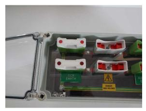
If the links are placed in the left position, then it can be clearly seen that the cables from the CCR to the Safety Isolation and Test Unit are connected to earth via the internal earth circuit. With the links in this position, the lid returned to the normal position, and a padlock fitted to the securing device then secure isolation and earthing has been achieved and the circuit cables within the CCR room/substation to be worked upon are at, or near, earth potential.
