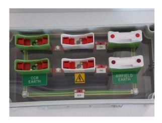
If the links are placed in the right position, then it can be clearly seen that the cables from the Safety Isolation and Test Unit out to the Airfield lighting circuit are connected to earth via the internal earth circuit. With the links in this position, the lid returned to the normal position, and a padlock fitted to the securing device then secure isolation and earthing has been achieved and the airfield lighting circuit to be worked upon is at, or near, earth potential.
